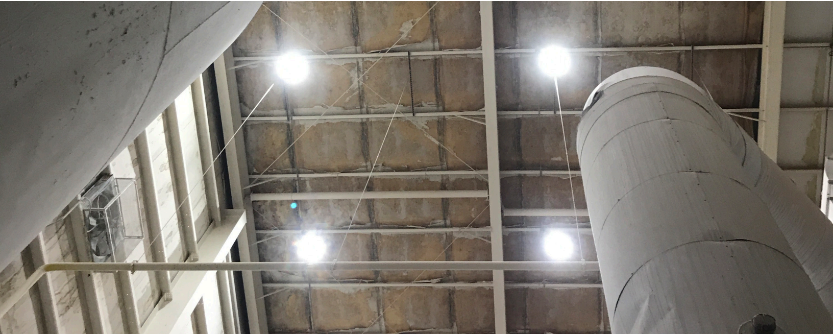
X2 150W FIXTURES SHOWN WITH TWIN MOUNT KIT AND ALUMINUM REFLECTORS
